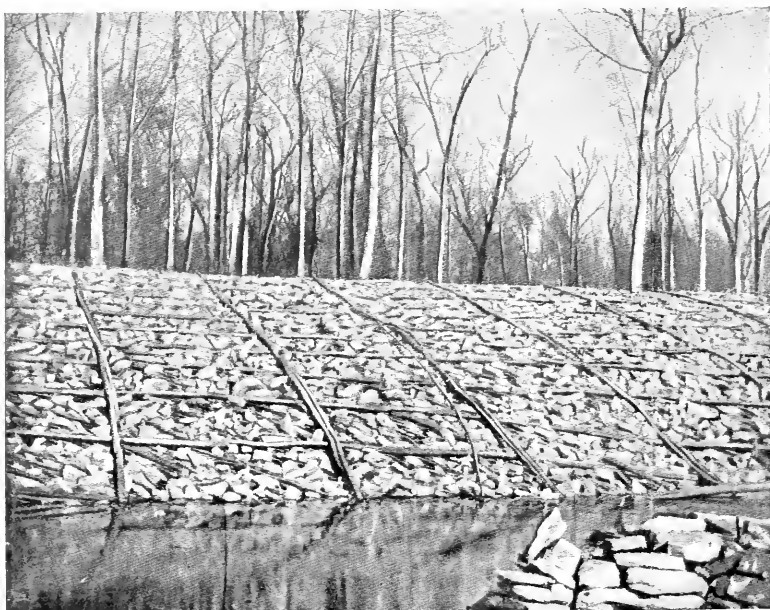
FINISHED BANK WITH POLE GRILLAGE AND STONE PAVING.
